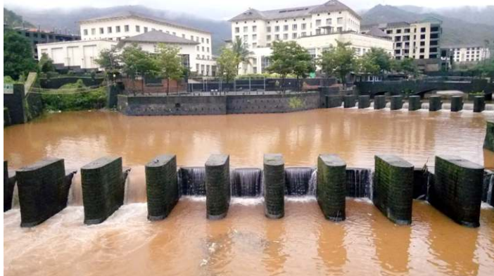
"Bridge over Valley of Krishna Godavari, Koyali River"
